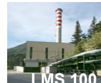
LMS 100 Bussi 110MW CIP6 repowering
